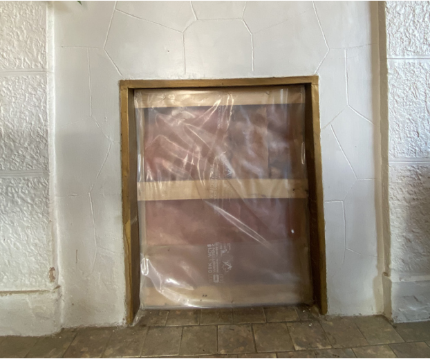
Sealing and insulating an unused chimney. | Jacob Ulickij
