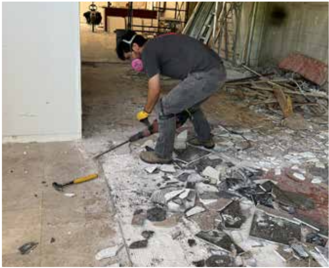
Left: The space at Nuestra right after Antonio and Nichola took possession. Centre: The space at Nuestra stripped down to the studs with all the tile and marble samples still on the floor. Right: Jackhammering the sample tiles off the floor mid-renovation.
