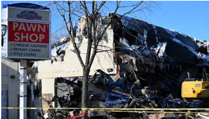
The Avenue Trading Post was destroyed by a fire and then demolished into a pile of rubble two days later. | Steven Michos
