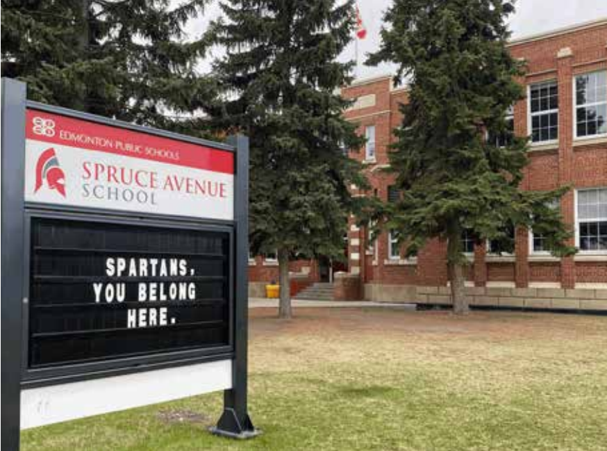
Spruce Avenue School, located on 114 Avenue and 102 Street, was built in 1928. The old red brick building holds historic significance for many in the community | Mikayla Pohl
