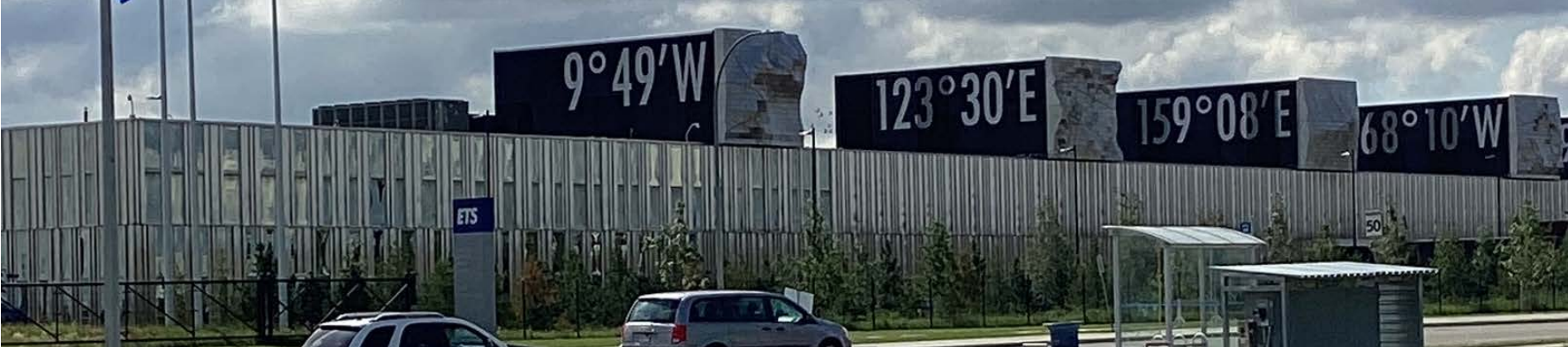
Five rooftop sculptures top the stainless steel cladding of the Kathleen Andrews Transit Garage on Fort Road, just north of the Yellowhead Highway (Highway 16). | Constance Brissenden
